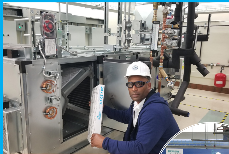
▶ Above, A Student in The Building Automation Systems Technology Program Replacing the Air-Conditioning Filter for Large Building
